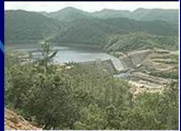
Challilo SHP Project in Belize under construction
